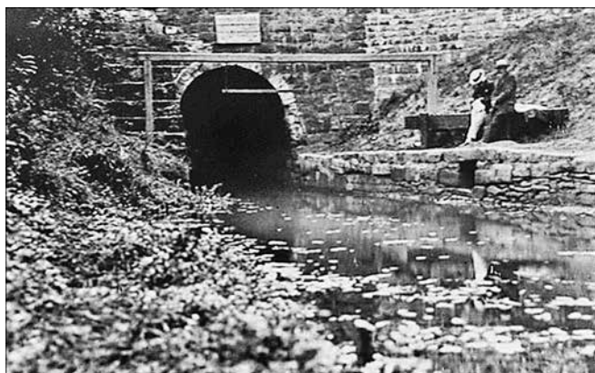
The east portal of Butterley Tunnel
